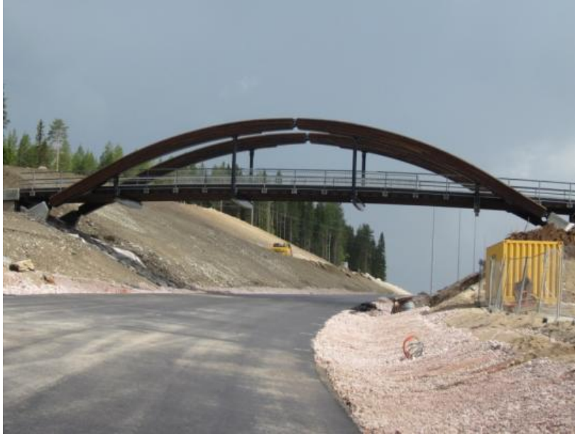
Figure 4. Dual copper/creosote treated glulam in the Åset Bridge in Norway, built 2014.
