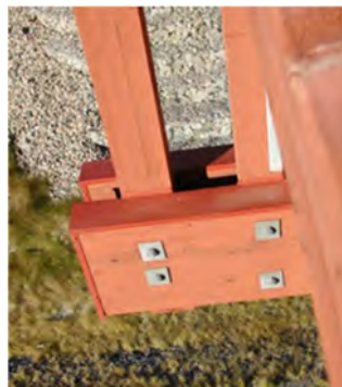
Figure 5.20. Good design, steel cover on horizontal surface and end grain of glulam crossbeam.
