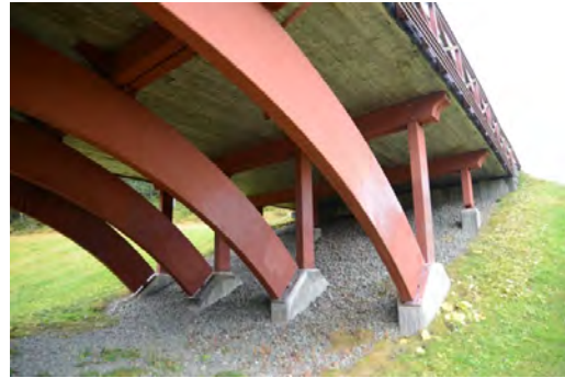
Figure 5.4. Good design, ground is covered with gravel (and the grass is cut).
