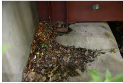
Figure 6.5. Dirt and old leaves on the concrete foundation
