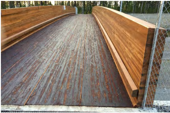
Figure 4.32 Longitudinal glulam deck.
