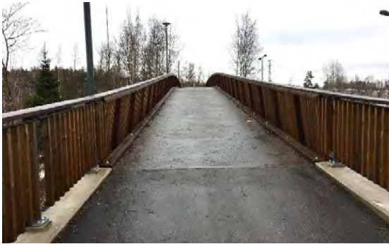
Figure 4.1 Asphalt cover on the timber deck
