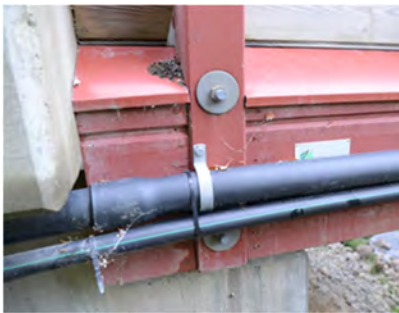
Figure 5.15. Bad detail, many constructions are problematic to inspect both due to accessibility and to installations attached afterwards, for example cables on the outside of deck panel that make it very difficult to control bar forces.
