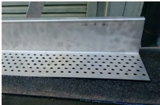
Figure 4.19. Steel angle with perforations in horizontal leg
