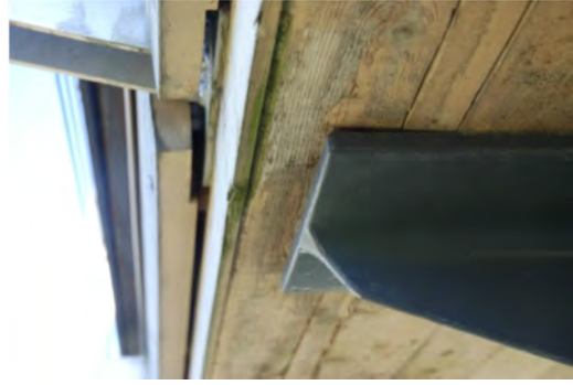
Figure 5.12. Good design, a small drip nose prevents water coming on the side of the deck to drain further under the deck. Drip nose and pulled in cross-member can reduce moisture invasion in deck.
