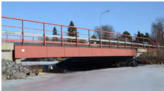
Figure 3.1 Stress-laminated plate bridge, span 17 m, Lövosundet, Holmsund, Sweden
