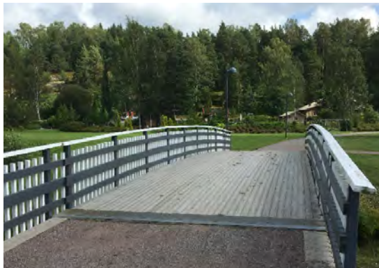
Figure 4.2 Longitudinal nailed plank deck
