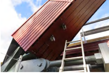
Figure 5.28. Good design with cladding. Moisture sensors have been installed for control at the bottom part of the arch where there is the largest risk of moisture.
