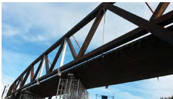
Figure 1.2 Construction of timber truss bridge, Norway
