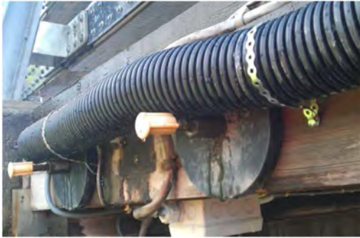
Figure 5.13. Bad detail, cables mounted afterwards are placed on the outside of the wooden deck without regard to the structure and they will moisten the wood.
