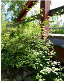
Figure 5.3. Bad detail, too much vegetation near the bridge end.
