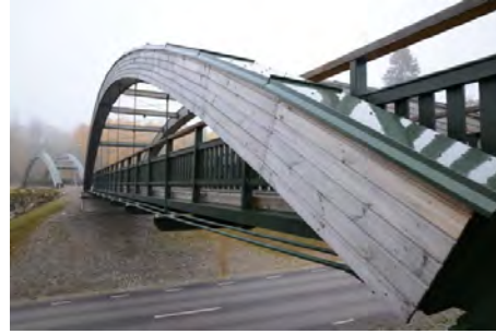
Figure 5.29. Good design with cladding of untreated wood and steel cover on top.
