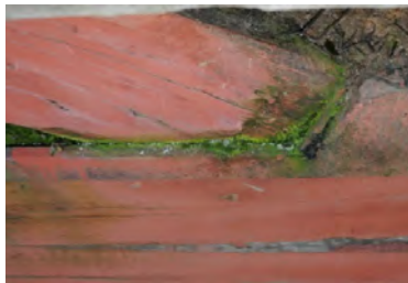
Figure 6.6. Growth of moss at connection
