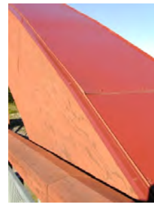
Figure 5.27 Arch bridges. In A the arch was unprotected but painted and had several cracks. In B the top of the arch was protected with a steel cover, but the sides were still unprotected. In C the sides were covered with a ventilated cladding of painted plywood sheets. The growth of cracks should then be significantly reduced and water cannot penetrate into the cracks.
