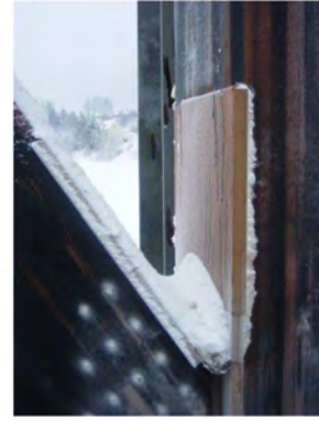
Figure 5.26. Good design, metal fitting protects the slot.
