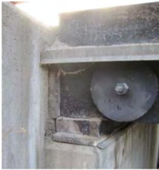
Figure 5.7. Bad detail, sill beam protrudes outside deck.
