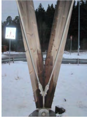
Figure 5.24. Bad detail, water can be concentrated to a slot between columns.
