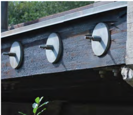
Figure 4.16. Creosote impregnated deck edge
