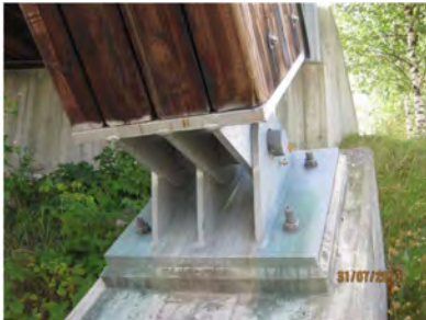
Figure 5.30. Bad detail, copper ions from copper fitting runs down to the underlying joint and corrodes the zinc coating.
