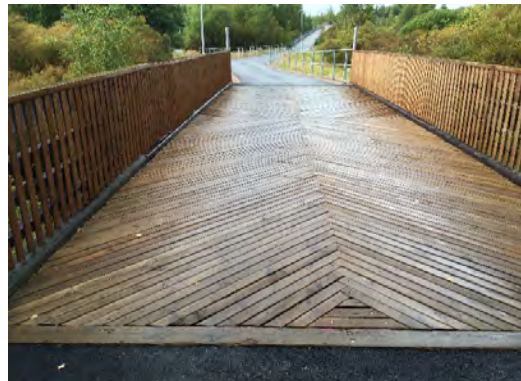
Figure 4.3 Diagonally nailed plank deck
