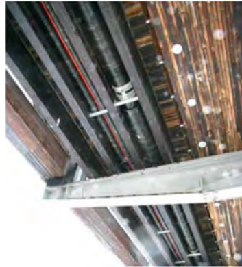
Figure 5.14. Good design. Cable duct laid over transverse beams between longitudinal beams for the sidewalk.
