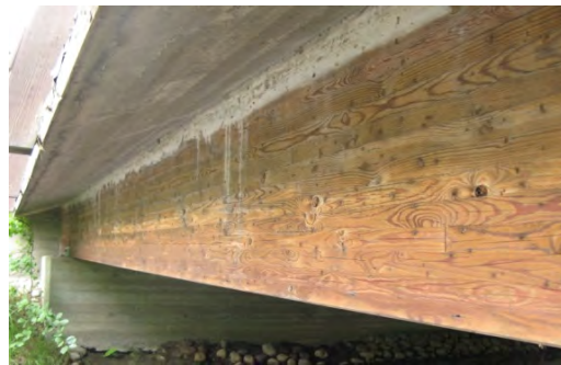
Figure 3.13 Timber beam and concrete slab
