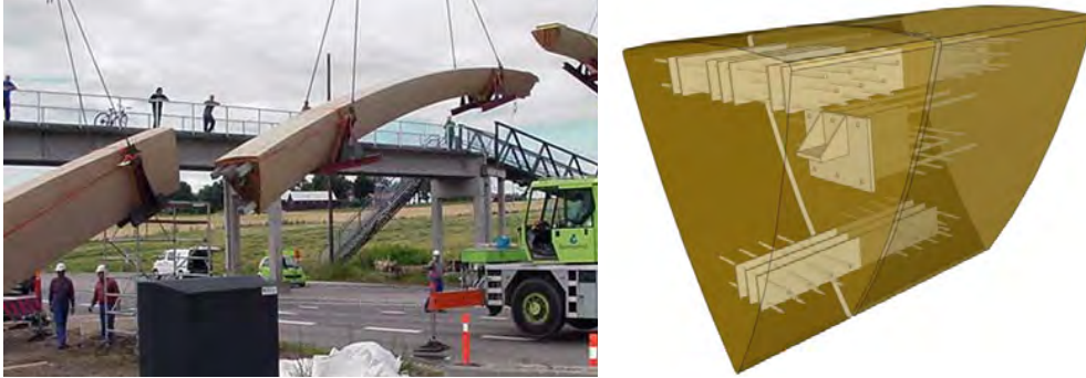
Figure 3.54 Leonardo Footbridge (2001), Norway, left: the central arch under assembly, right: visualisation of the splice joint
