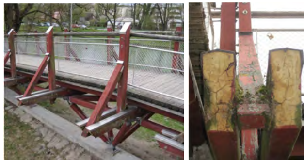
Figure 5.33. Bad detail, railing with some constructive protection (covering of horizontal parts), but connections between parts prevent adequate ventilation.
