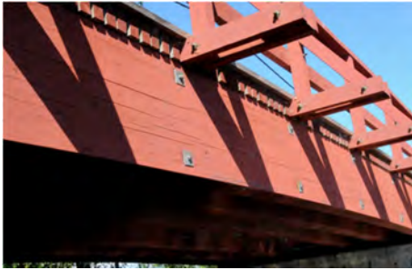
Figure 6.4. Painted glulam beam with some cracks
