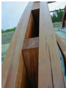
Figure 5.27 Arch bridges. In A the arch was unprotected but painted and had several cracks. In B the top of the arch was protected with a steel cover, but the sides were still unprotected. In C the sides were covered with a ventilated cladding of painted plywood sheets. The growth of cracks should then be significantly reduced and water cannot penetrate into the cracks.
