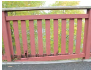
Figure 6.7. Rot in lower part of railing
