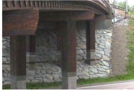
Figure 5.2. Good design, ground has good covering to avoid vegetation.
