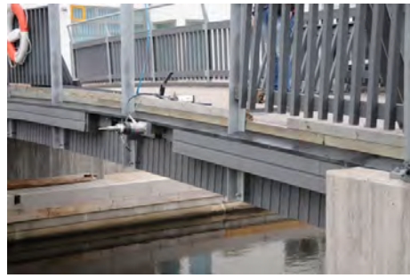
Figure 5.16. Good design, the cladding can easily be removed to control the bar forces and optionally for restressing the bars.
